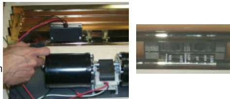
Blower switch box slides into bottom louver assembly and is screwed into place. Place label on outside of louver as shown.
